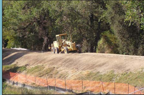
Levee embankment grading
