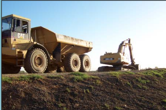
Hauler and excavator on levee crown
