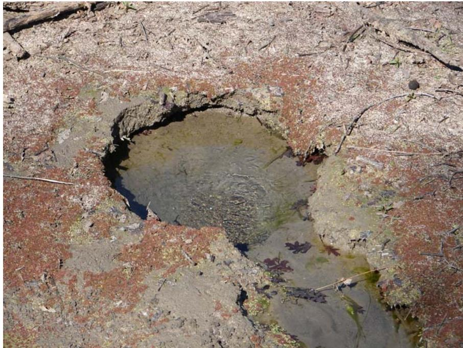
Photograph No. 2: Close-up of Boil in Pritchard Lake Intake Canal (03-04-08)
