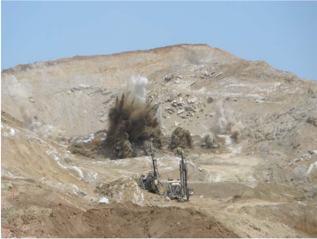
View of rock blasting in the spillway excavation
