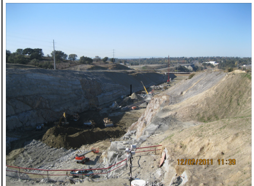
Ongoing excavation of downstream end of Control Structure.
