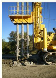
◀ Deep Soil Mixing rig installing cut off wall ▲ New levee at Garden Hwy and Sankey Rd.
