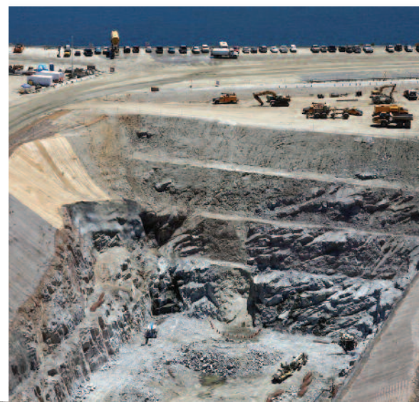
(Left) Improved levees on east side of Natomas Basin. (Right) Excavation of auxiliary spillway at Folsom Dam.
