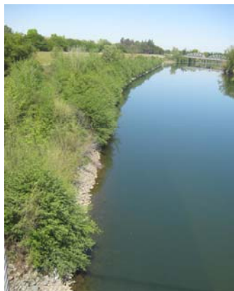
Bank Protection Project on the American River at CSU, Sacramento
