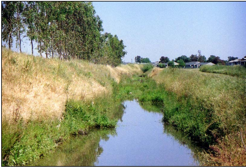
Figure 1 - Old, channelized section of Robla Creek prior to construction of RLCCA
