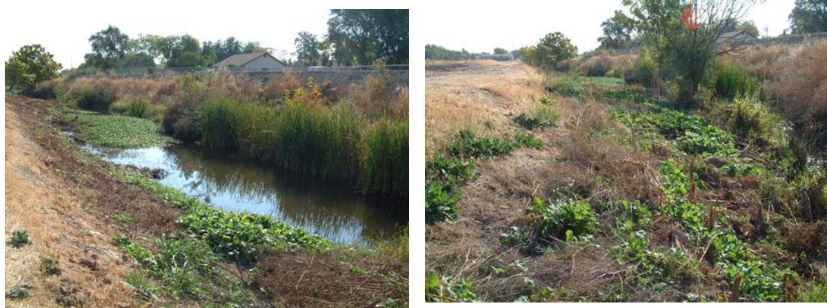
Figure 1 – Old Section of MCDC Prior to Construction
