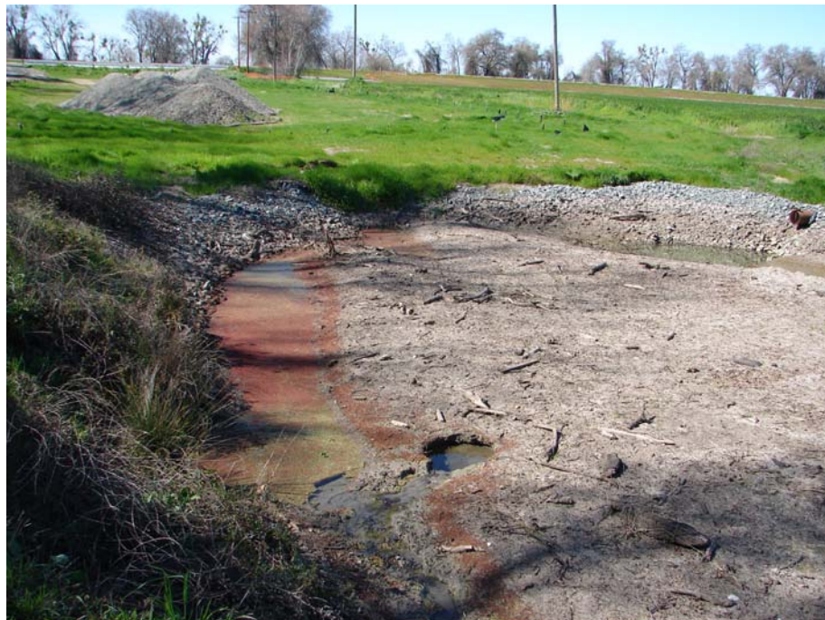
Photograph No. 1: Boil in Pritchard Lake Intake Canal (03-04-08)
