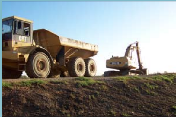
Hauler and excavator on levee crown
