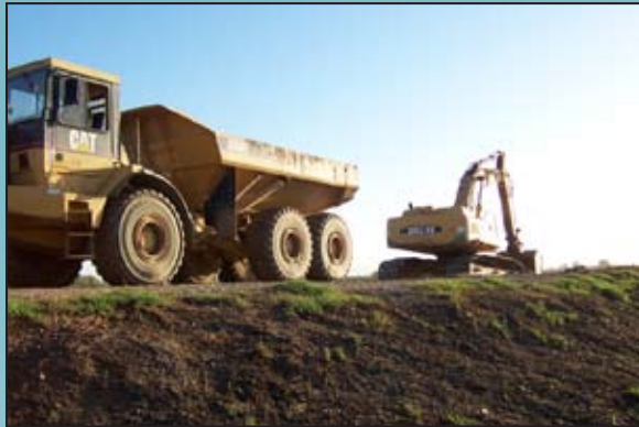
Hauler and excavator on levee crown
