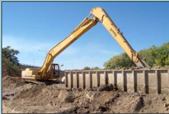
Construction of a slurry cutoff wall
