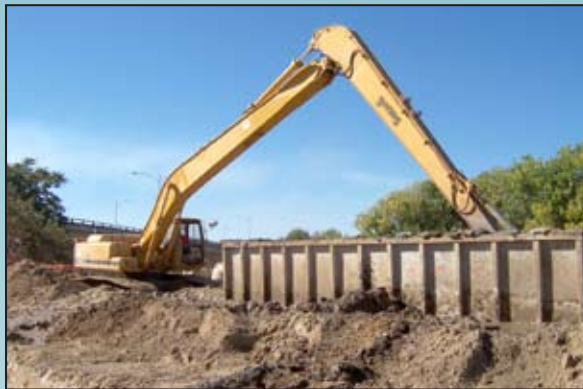
Construction of a slurry cutoff wall
