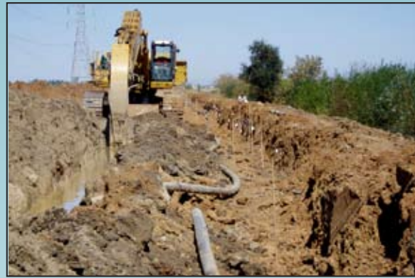
Construction of a slurry cutoff wall
