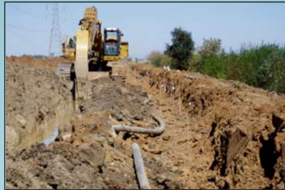
Construction of a slurry cutoff wall
