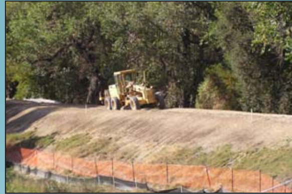
Levee embankment grading
